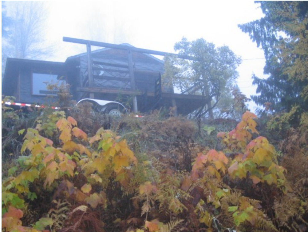
Figure 2. Photograph showing wooden siding and open decks.
